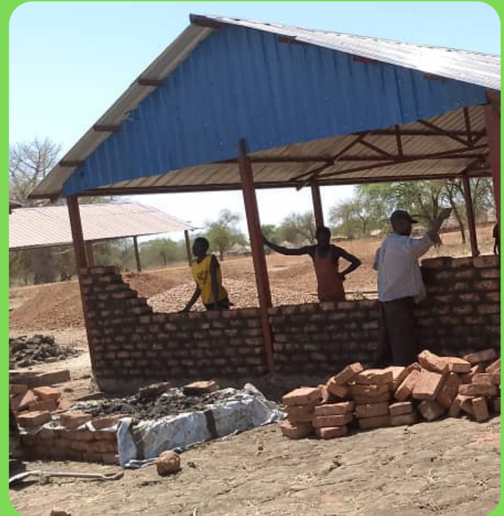
ECD AND PRIMARY SCHOOL BUILDING UNDER CONSTRUCTION
